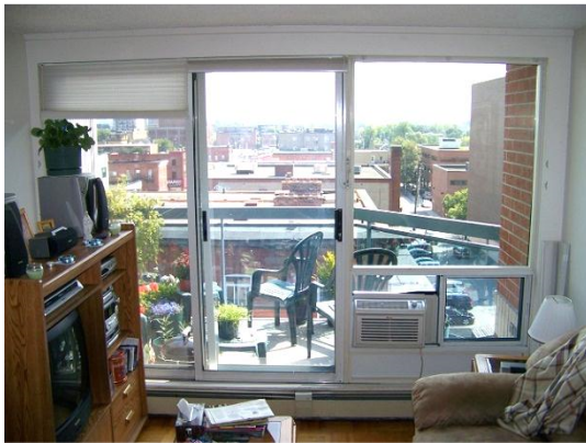
Figure 3: Test building, HSG apartment living room. Typical arrangement of sliding patio door and fixed-over-slider window, with balcony beyond.
