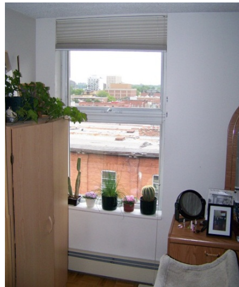
Figure 4: Test building, HSG apartment bedroom. Typical arrangement of awning-over-fixed window.
