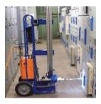
Roll-up Racking with Full Breaker Removal Tools: Variations on roll-up style may be equipped with an extraction type mechanism for breaker insertion and removal in conjunction with jack accessories to lift and transport a large circuit breaker. For large medium voltage and heavy air frame circuit breakers, varieties can also incorporate a crane for hoisting and support for these heavier circuit breakers.
