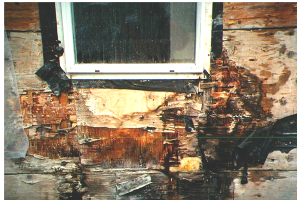
Figure 7: Example of sheathing damage due to rain penetration at window sills
