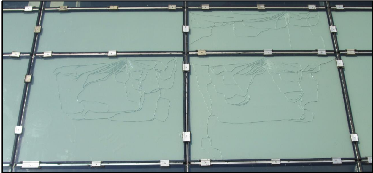
Figure 1 – Example of Glazing Failures Attributed to Thermal Stress in Spandrels Insulating Glazing Units
