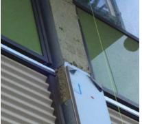
An example where the assembly Uvalues might be fine when thinking in parallel but the overall thermal performance is poor because of thermal bridging at interface details
