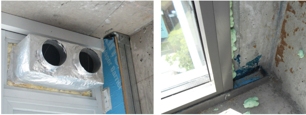
Figure 7: Careful thought in 3D is required to ensure continuing of air and water leakage control.
