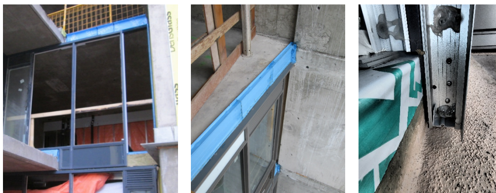
Figure 2: Canadian window wall system during installation. Left, story high panels have been installed with the other half of the frame extended to cover the floor slab.
