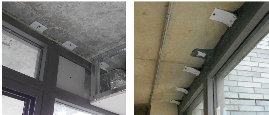
Figure 3: Examples of strap anchors at the head rail of a window wall. Left, straps secured with concrete screws to the underside of the floor slab with one component polyurethane foam air sealant foam in the rough opening gap as an air seal. Right, rough opening gap exceeds the length of the strap so straps are extended by stitching end-to-end. A gunned sealant was applied over the foam to ensure continuity of the air barrier. Encapsulating the perimeter of the straps may be needed if access behind the strap for sealant application is restricted.
