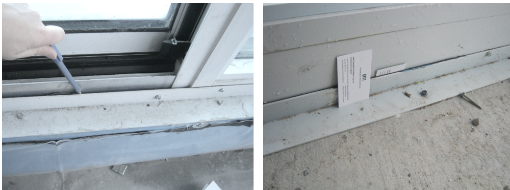
Figure 6: Careful thought in 3D is required to ensure continuing of air and water leakage control.
