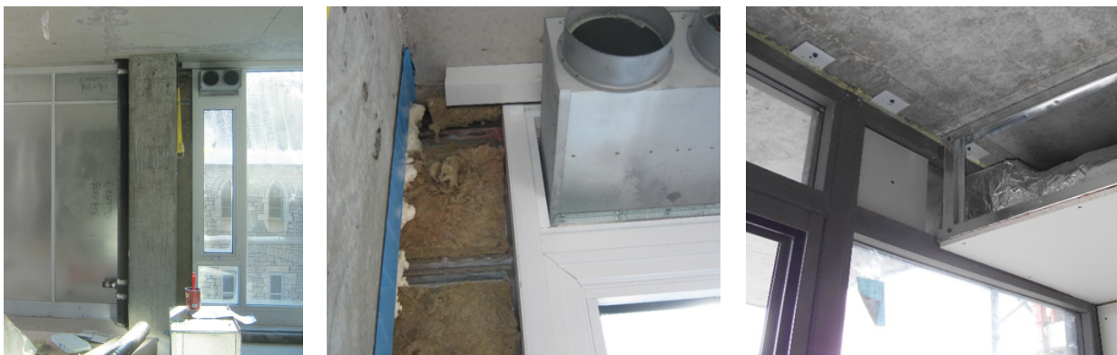
Figure 4: Examples of interference/lack of coordination between structure, mechanical services and window wall systems.
