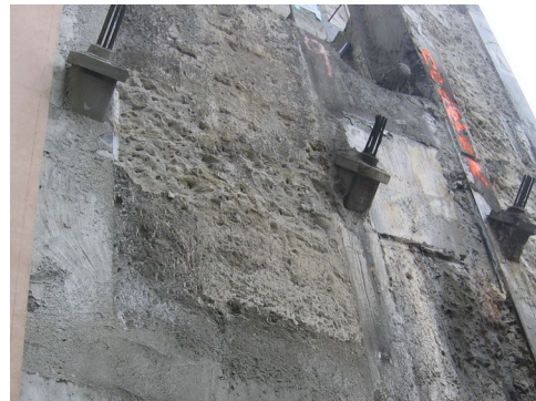
Image 3 – Sample of CSM shoring wall prior to being prepared as bentonite substrate
