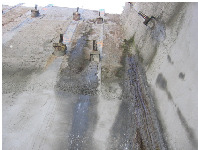
Image 2 – Water seepage through CSM wall at tie backs
