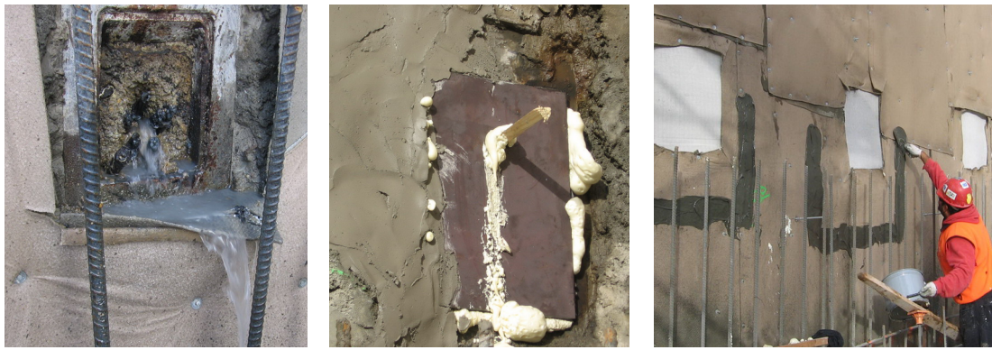
Image 3 – Tie Back removal, capping to prevent water seepage and bentonite patching over tie backs
