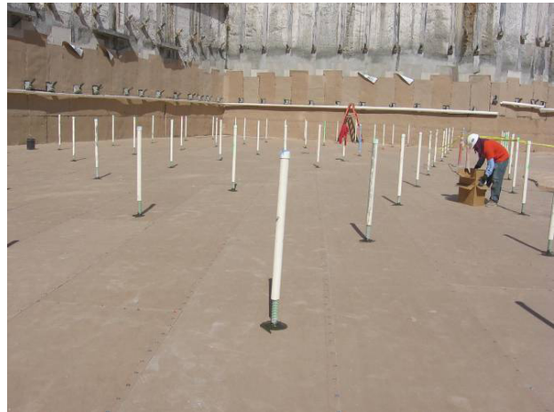
Image 1 – Bentonite waterproofing membrane installed over rat slab and sealed around tie down penetrations
