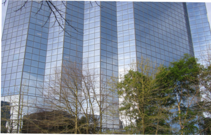
Figure 1. This building has a 100% glazed wall, but 50% of the wall area is vision glass (reflective and transparent) and 50% of the area is spandrel glass (reflective and opaque).
