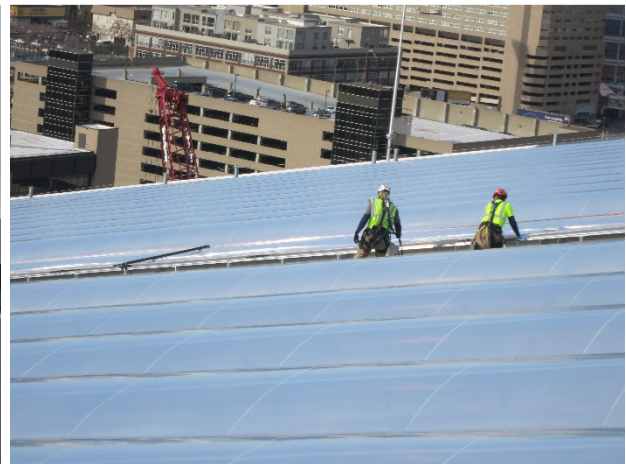
Figure 20- Installation of ETFE cushions
