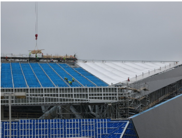
Figure 19- Installation of ETFE cushions
