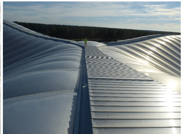
Figure 14- ETFE roof system from exterior
