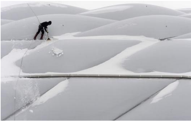
Figure 9- Manual removal of snow from an ETFE system
