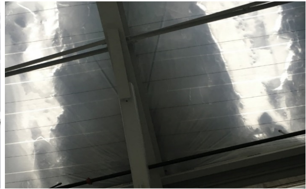
Figure 10- An ETFE system in a deflated state, supported by snow cables, with snow load
