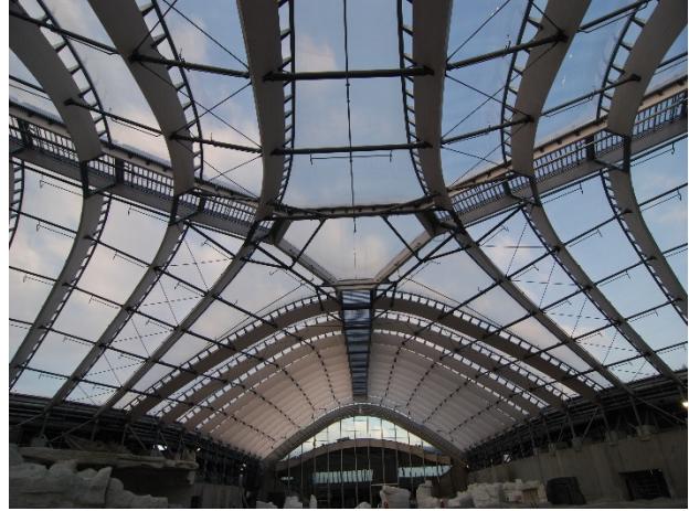
Figure 16- ETFE roof system from interior
