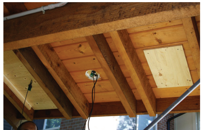
Figure 7 Control assembly sensors.
