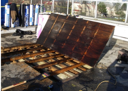
Photo 3 Investigation of Damaged Roof Sheathing before Roofing Renewal
