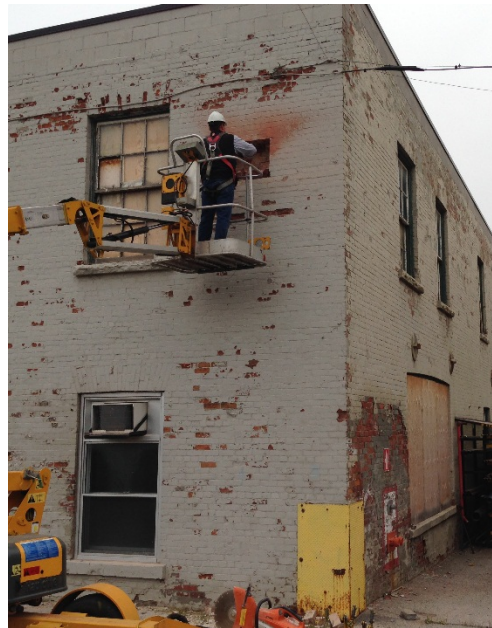
Photo 21 Investigation for a feasibility Study focused on evaluating the risks and benefits of insulating a brick masonry wall
