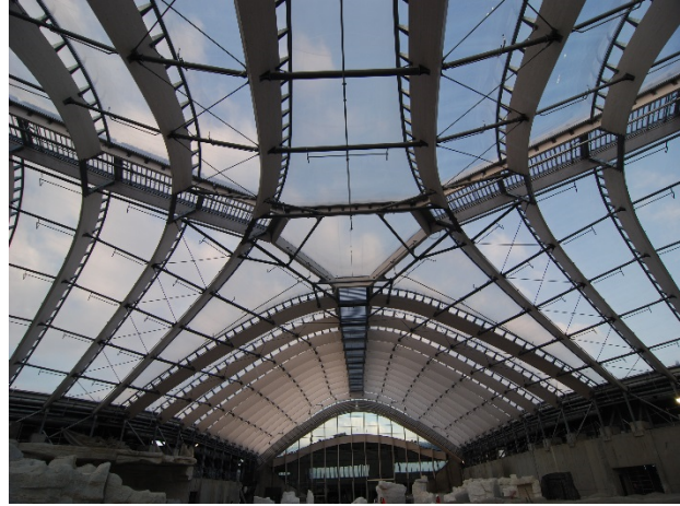
Figure 16- ETFE roof system from interior
