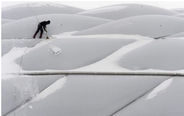
Figure 9- Manual removal of snow from an ETFE system Photo credit: SurfaceDesign
