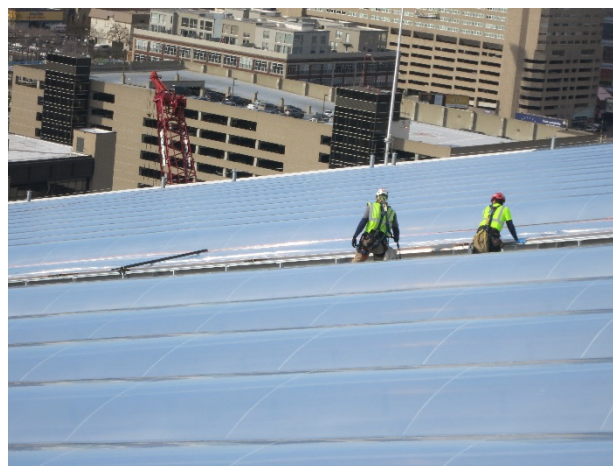
Figure 20- Installation of ETFE cushions
