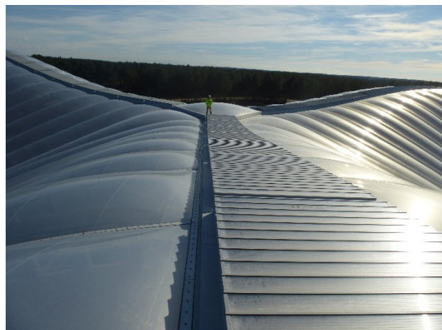
Figure 14- ETFE roof system from exterior
